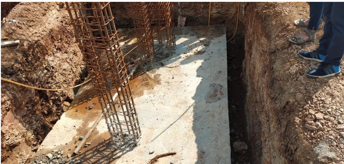
Combined Rectangular Footing with P.C.C.
