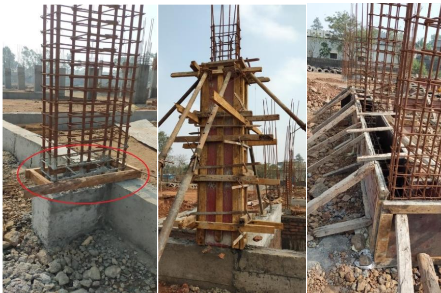
STARTER FORMWORK REINFORCEMENT
